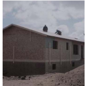
DTI Carpentry program participants work on roof.
